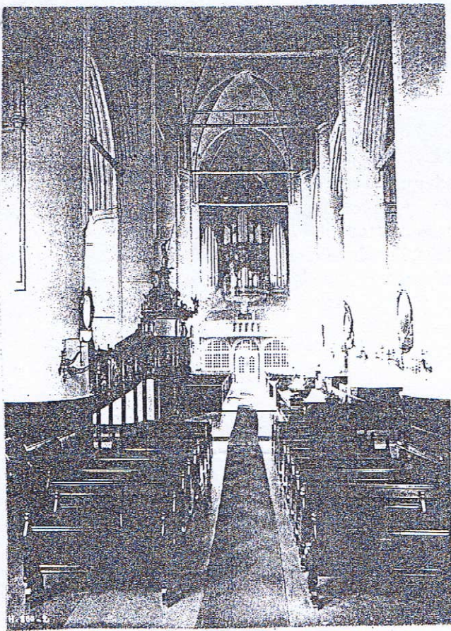
St. Catherine's interior view toward organ before its destruction Photo: Museum of City History, photo archives
